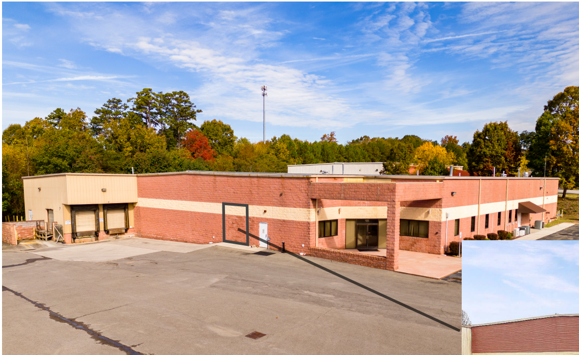
Recently installed drive-in door
