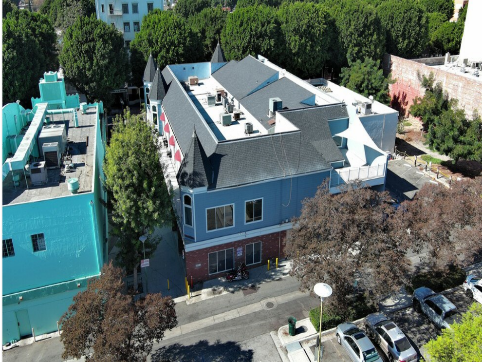
Side of Building
