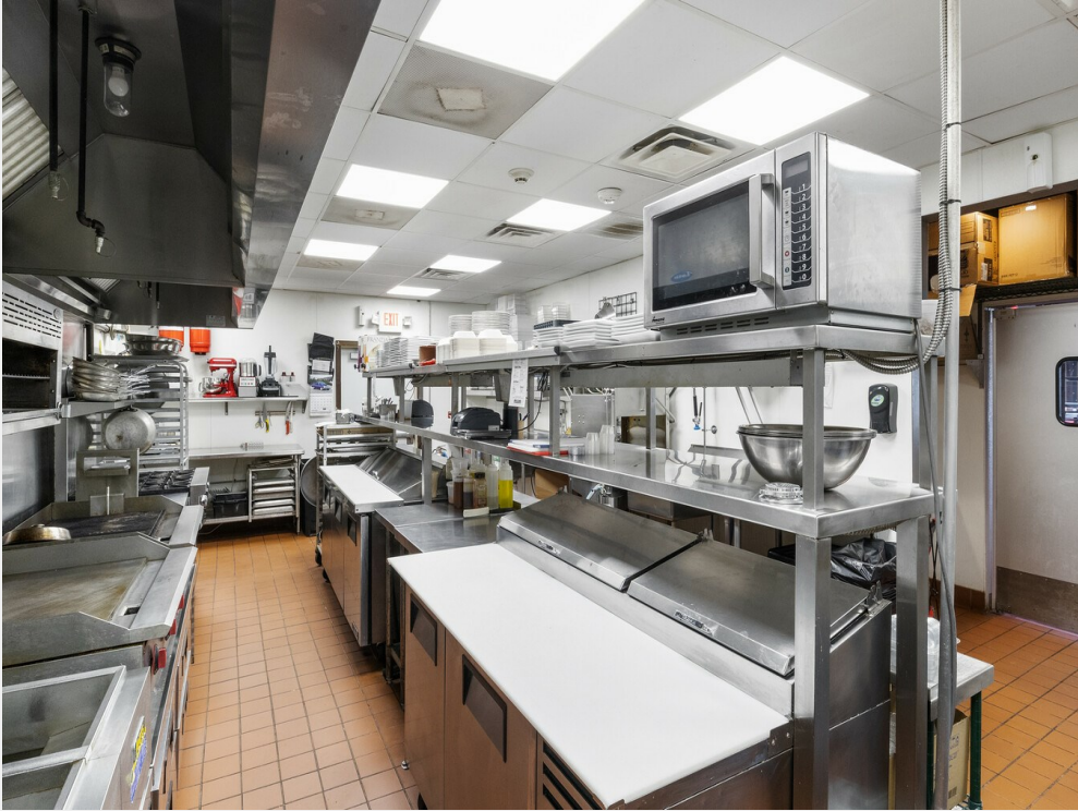
26-1289 Bagnell Dam Blvd - 26
