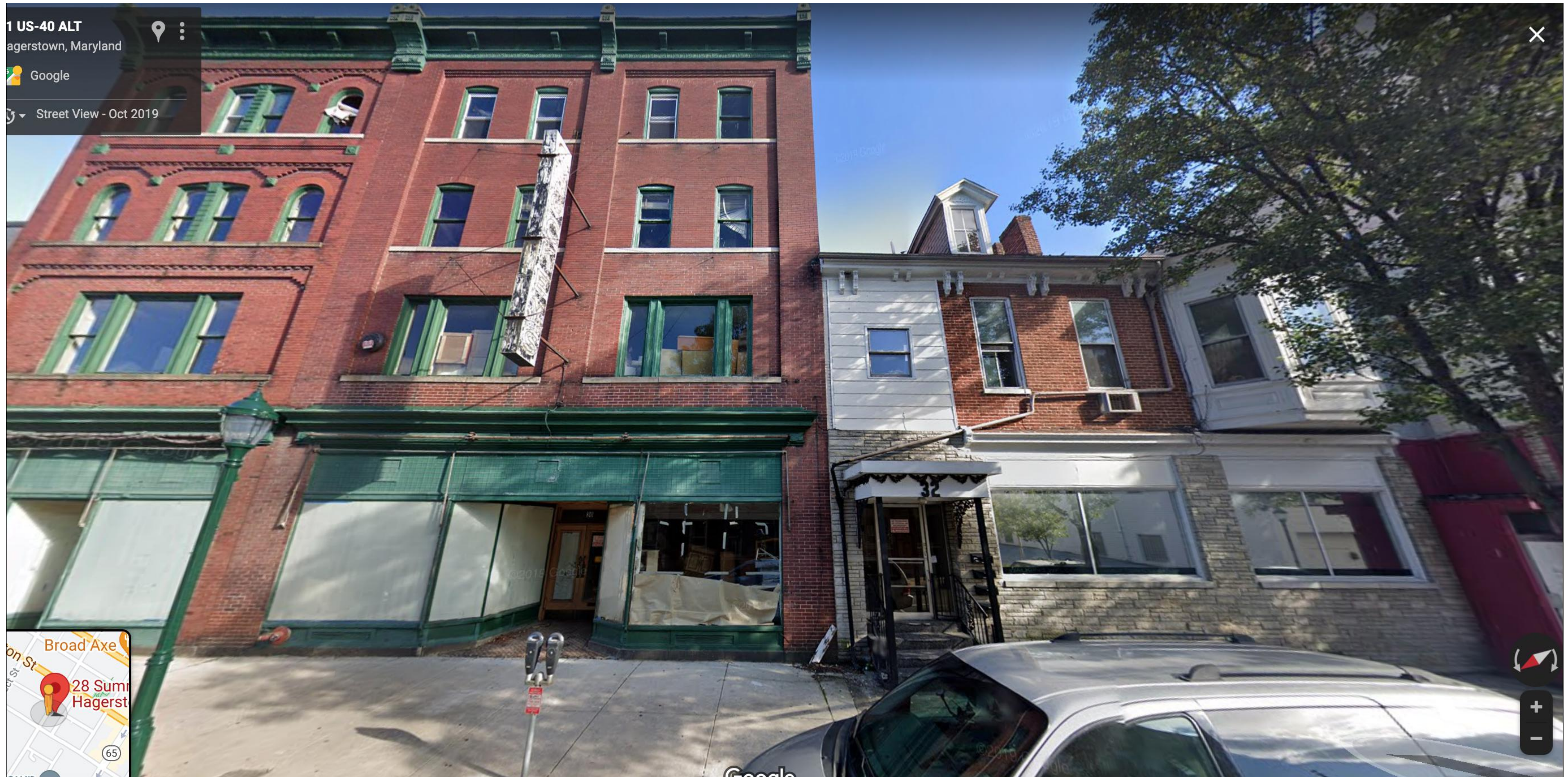
26-28-30 SUMMIT STREET (SHOCKEY BUILDING) EXISTING
