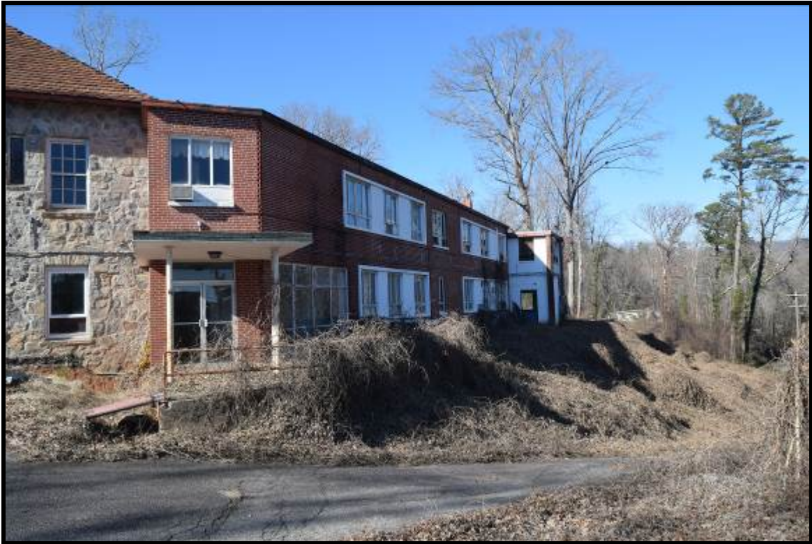
Photo 2: North wing addition to the hospital.
