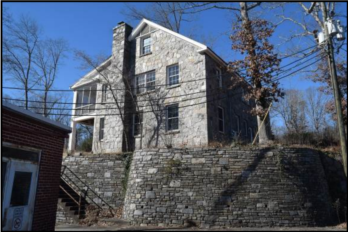
Photo 21: Stone residence on an adjoining parcel to the west of the south wing portion of the hospital.
