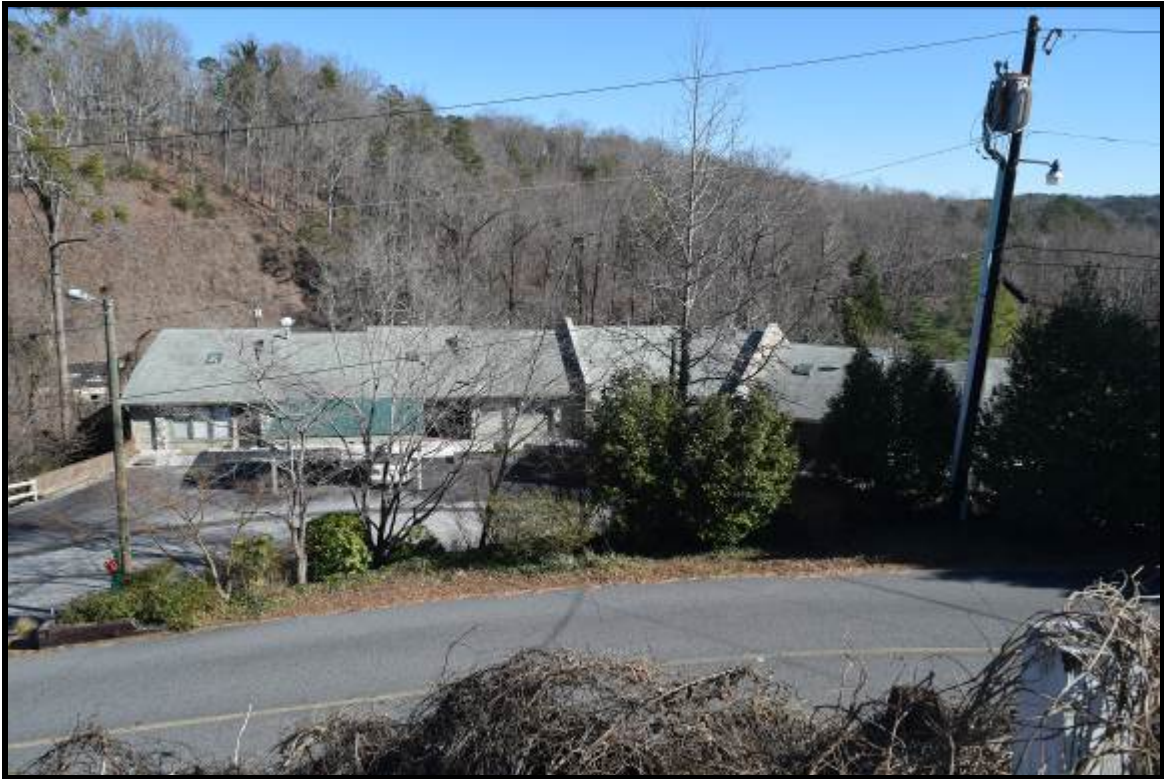
Photo 20: Commercial office building on the adjoining property to the east across Carolina Drive.
