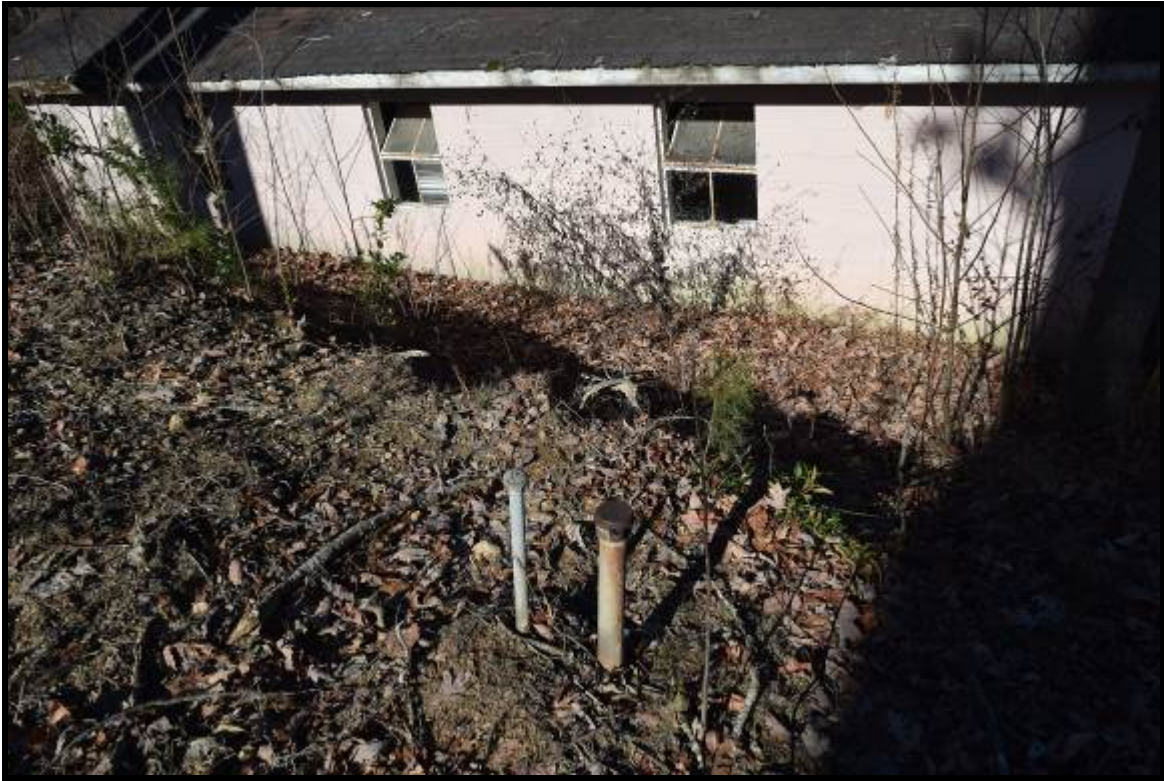
Photo 13: Vent pipe and fill pipe of heating oil UST (foreground) adjacent to the west side of the classroom building shown in Photos 11 and 12. The UST was found to be empty and is estimated to be approximately 300 gallons in capacity.
