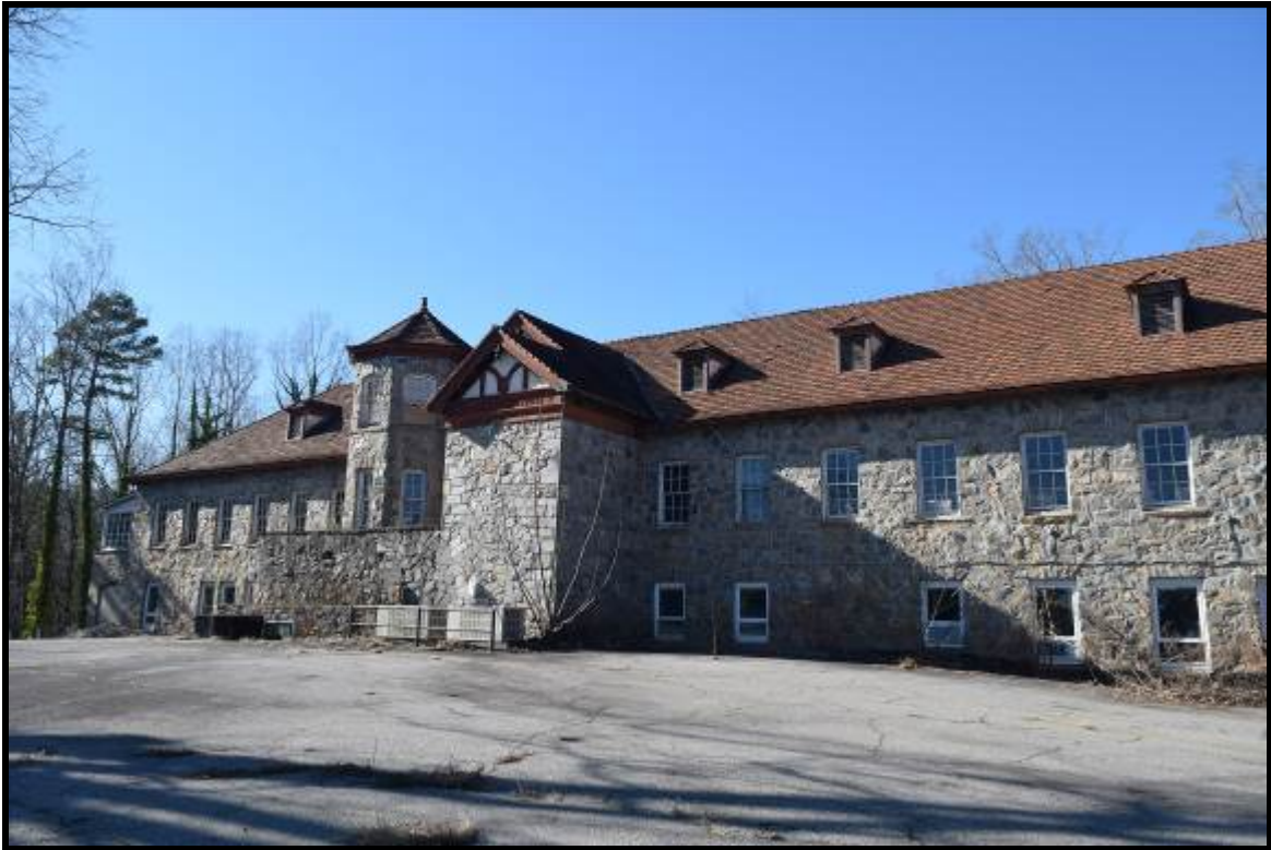
Photo 1: East exterior of original portion of the on-site hospital.
