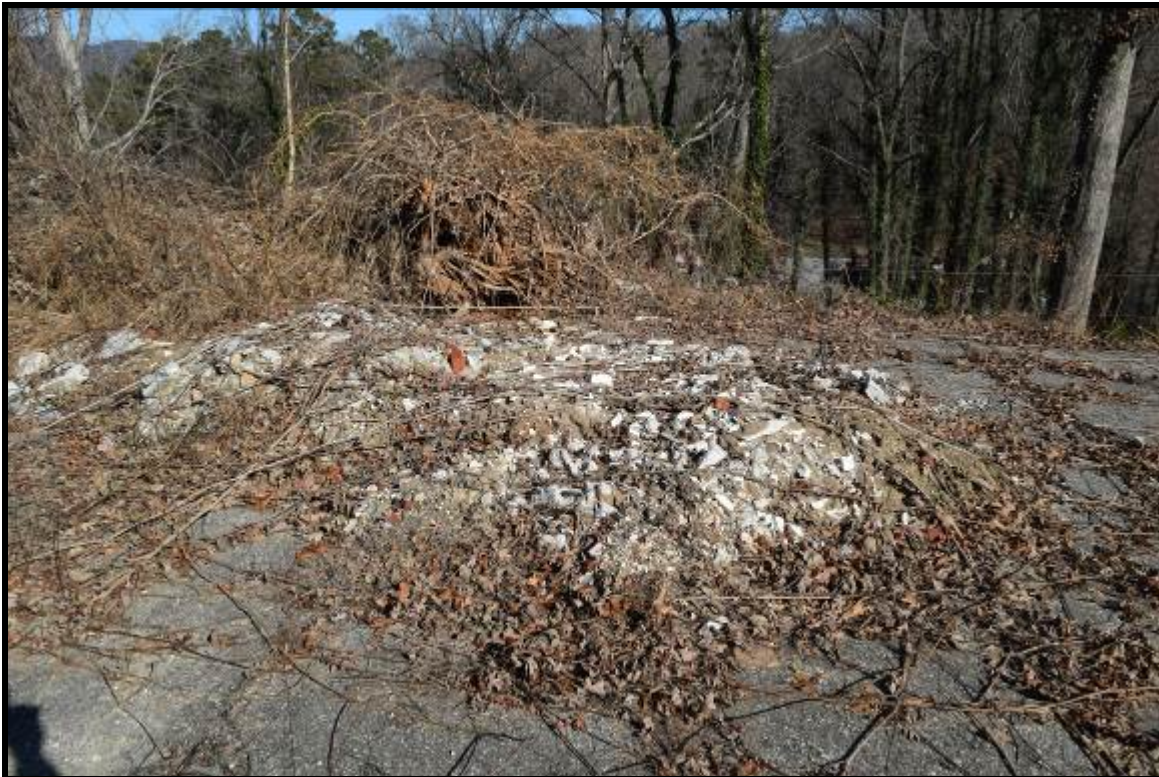
Photo 10: Piled debris at north end of west parking area. Debris appears to be associated with prior removal of interior areas. The debris pile may include asbestos-containing building materials.
