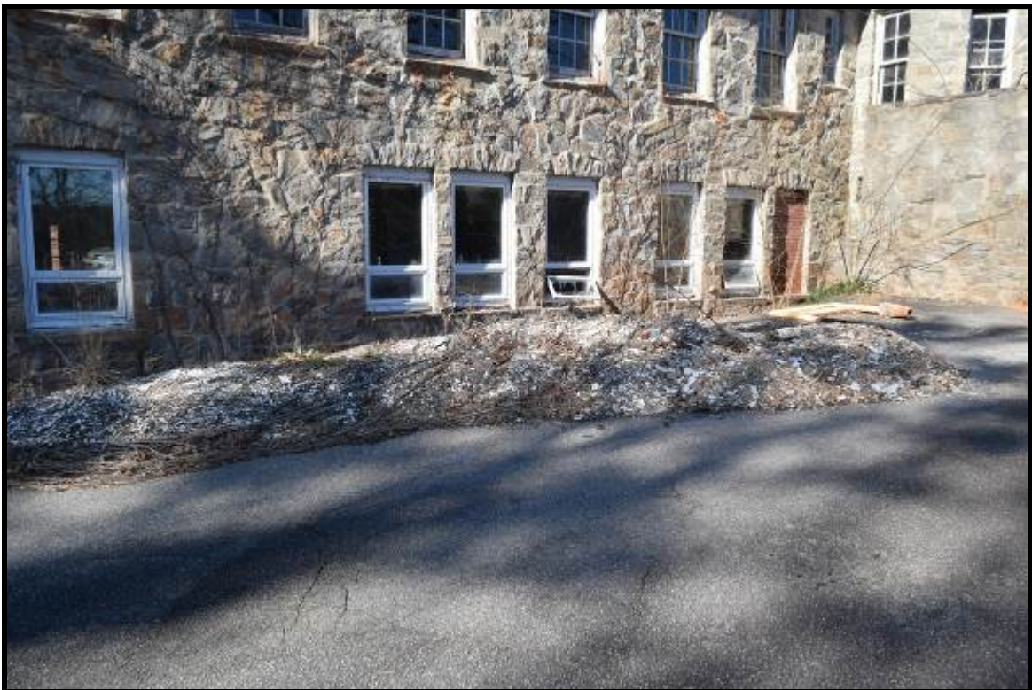
Photo 16: Debris pile adjacent to southeast corner of the original portion of the hospital. Debris appears similar to the pile shown in Photo 10.
