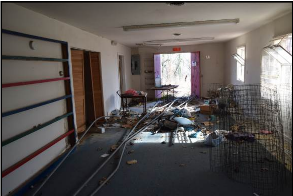
Photo 12: Interior of building shown in Photo 11.
