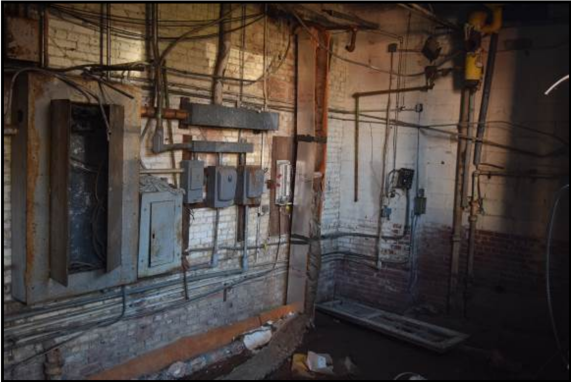
Photo 7: Boiler room (boiler removed) in the lower level of the hospital.
