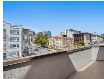
Multiple 3 rd Floor Exterior Balconies With City Views
