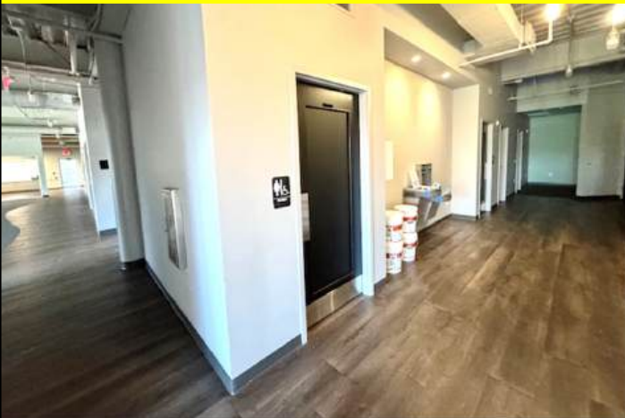
Restrooms/ Elevator Access
