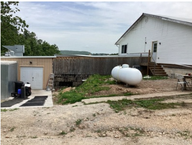
Rear of Kitchen
