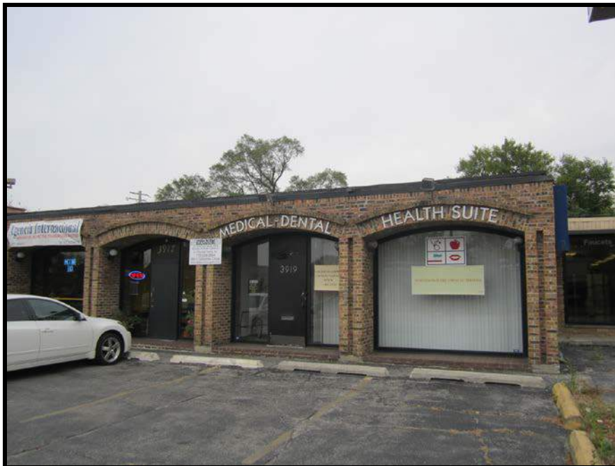
VIEW OF EASTERN ADJOINING PROPERTY
