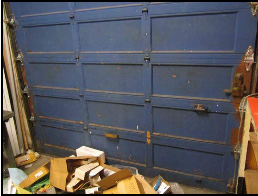
INTERIOR VIEW OF LOADING DOCK
