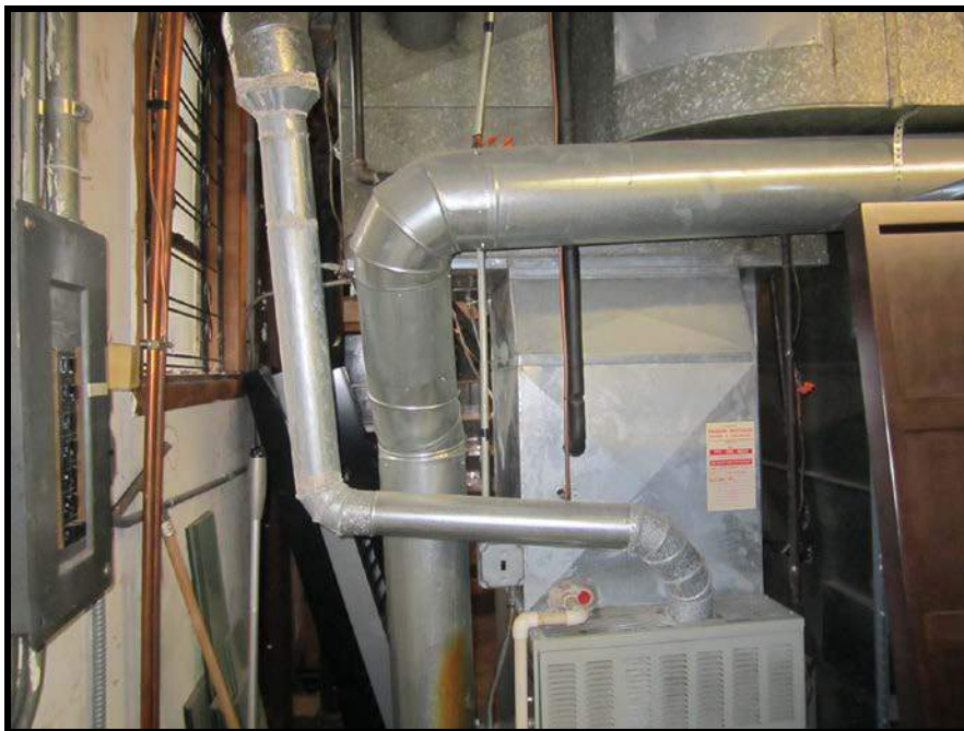
INTERIOR VIEW OF MECHANICAL AREA
