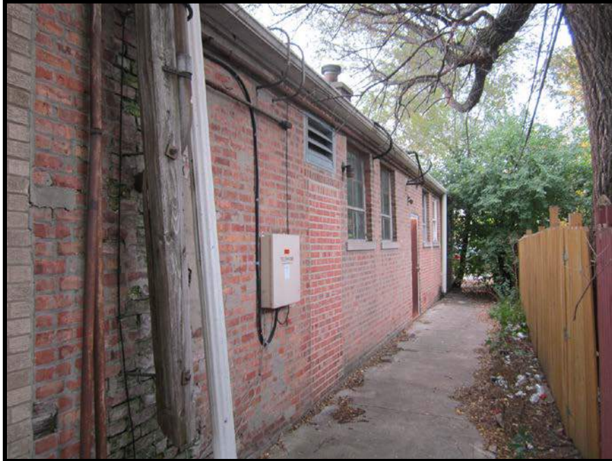
VIEW OF SUBJECT BUILDING'S SOUTH SIDE FACING EAST
