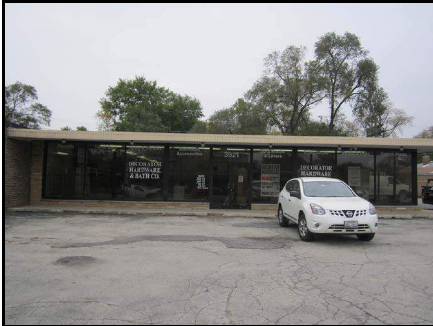
VIEW OF SUBJECT BUILDING FRONT FACING SOUTH
