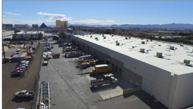
Grade & Dock Level Loading
