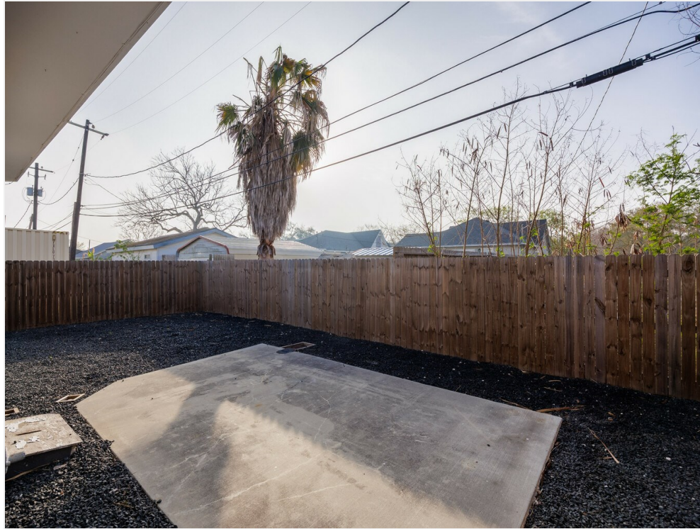
back of building
