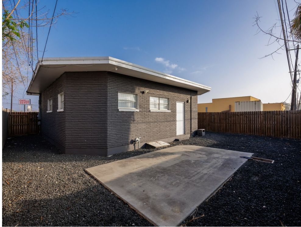
back of building
