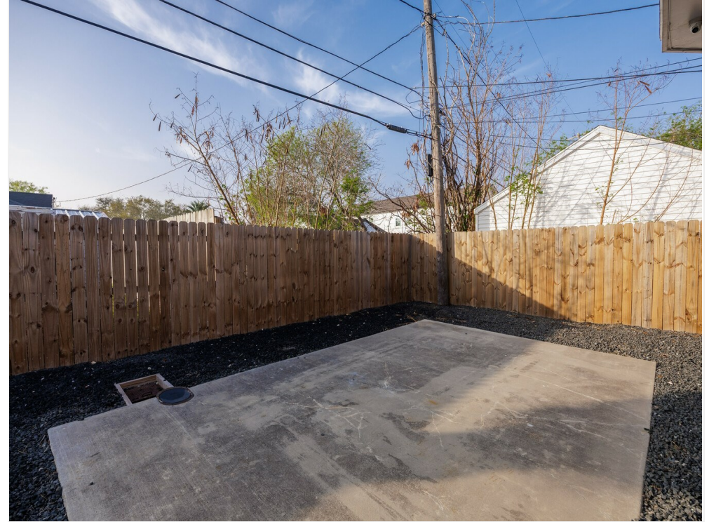
backyard cement pad
