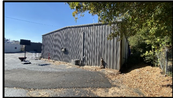
Typical Exterior View
