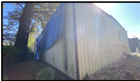
Typical Exterior View
