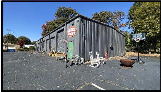
Typical Exterior View
