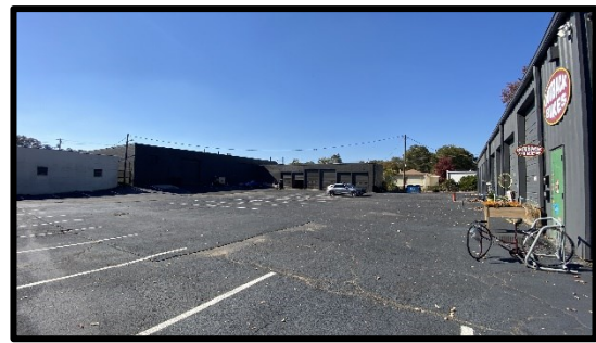
Typical Exterior View
