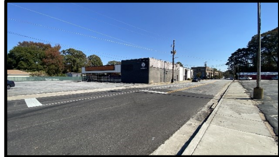
Typical Exterior View
