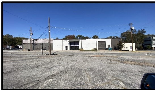
Typical Exterior View
