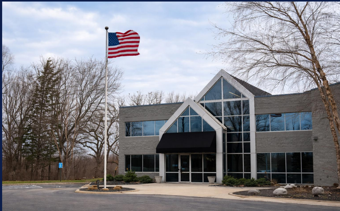
Front Entrance — South Elevation
