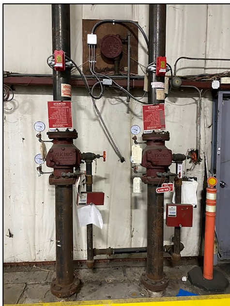
Sprinkler risers for wet system
