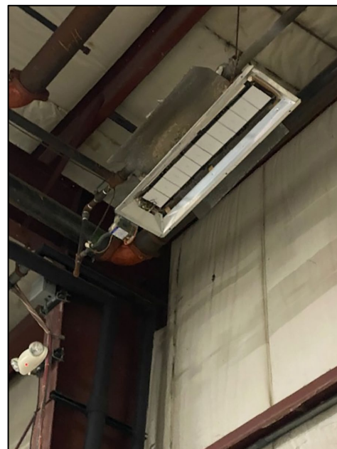
Gas radiant heat units throughout the building
