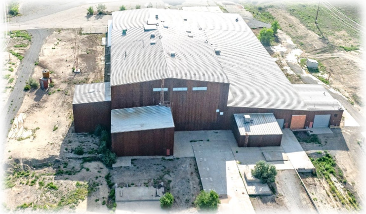
View of Facility facing East/Back of Building
