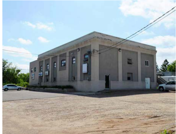
NW Corner of Building
