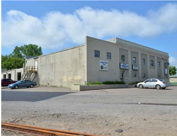
NE Corner of Building
