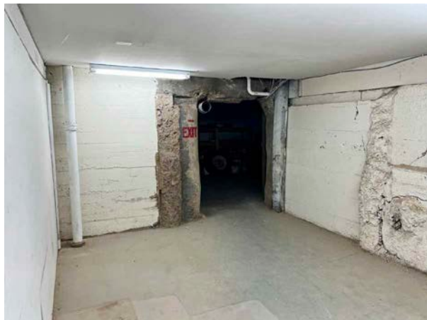
Vacant 100 - Lower Level Storage
