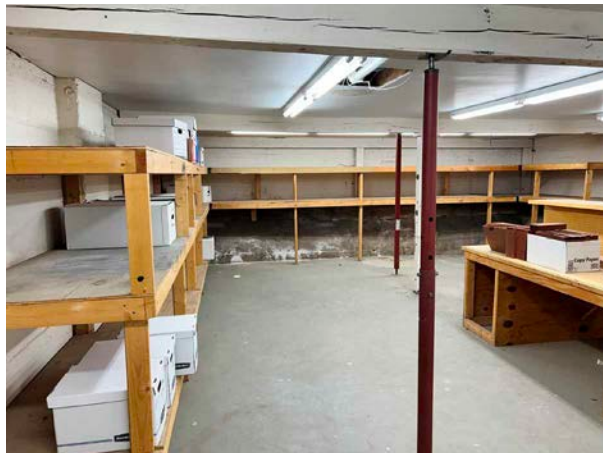
Vacant 100 - Lower Level Storage
