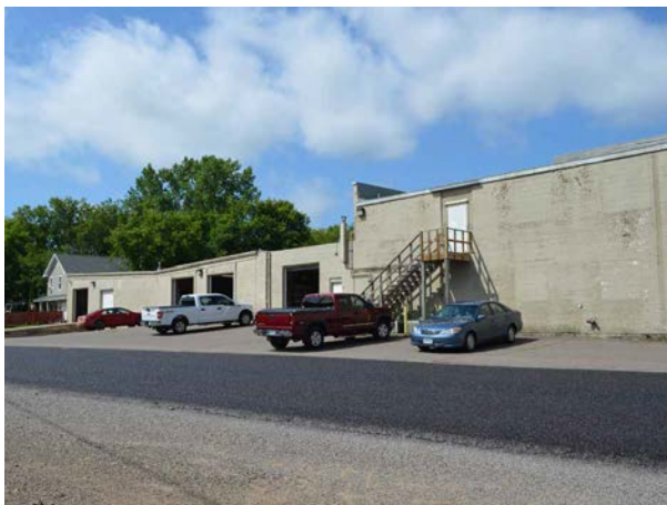
East Side of Building w/ OH Doors
