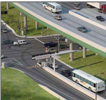
Northwest Corridor Express Lanes
