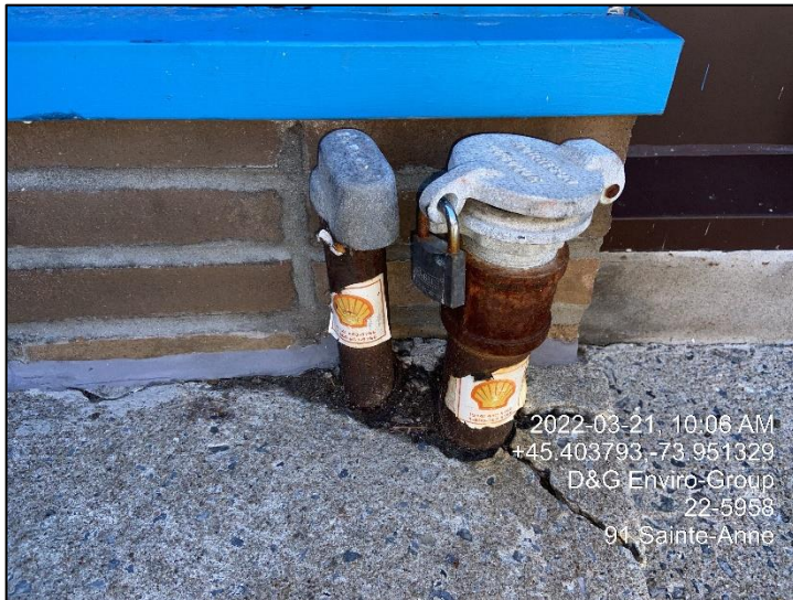
Photo 7 – Capped fill and vent pipes located on the northern exterior wall.
