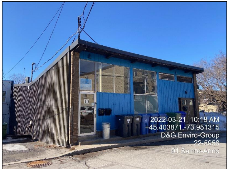
Photo 8 – Rear of the building.
