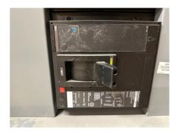
**Service: Service Disconnect Size** 800 AMP **System Ground:** System Ground Location
