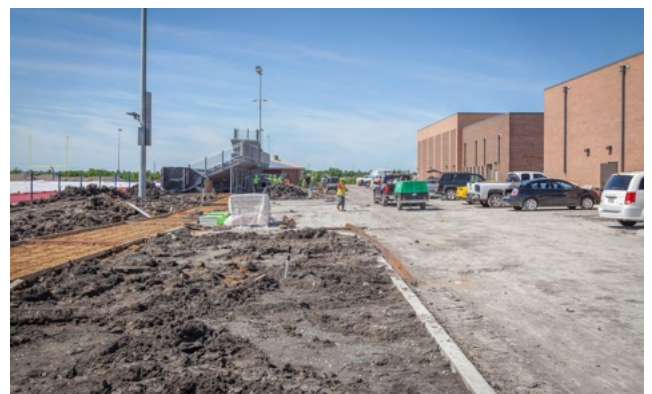
Construction of new middle school
