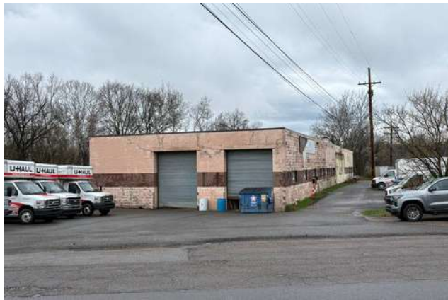
Front Elevation — Roll-Up Doors & Paved Lot
