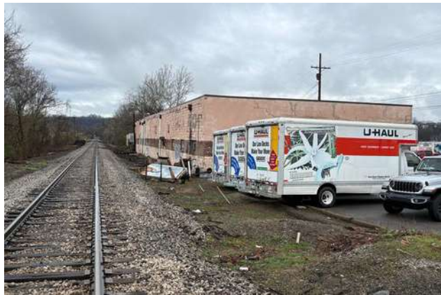
Rail Corridor View — Building Length & Rail Proximity
