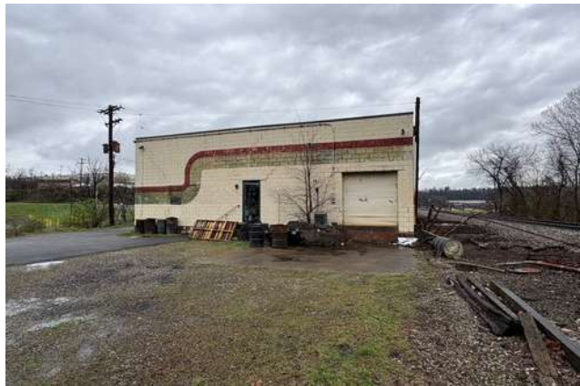
Rear Elevation — Adjacent to Active Rail Corridor
