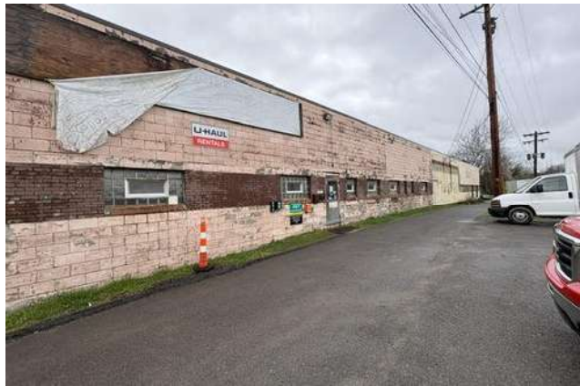
Street-Side View — U-Haul Signage & Access Drive
