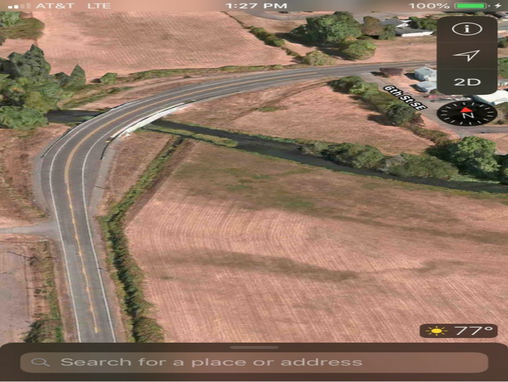
New High Clearance Wipper Road Bridge Crossing Mill Creek
