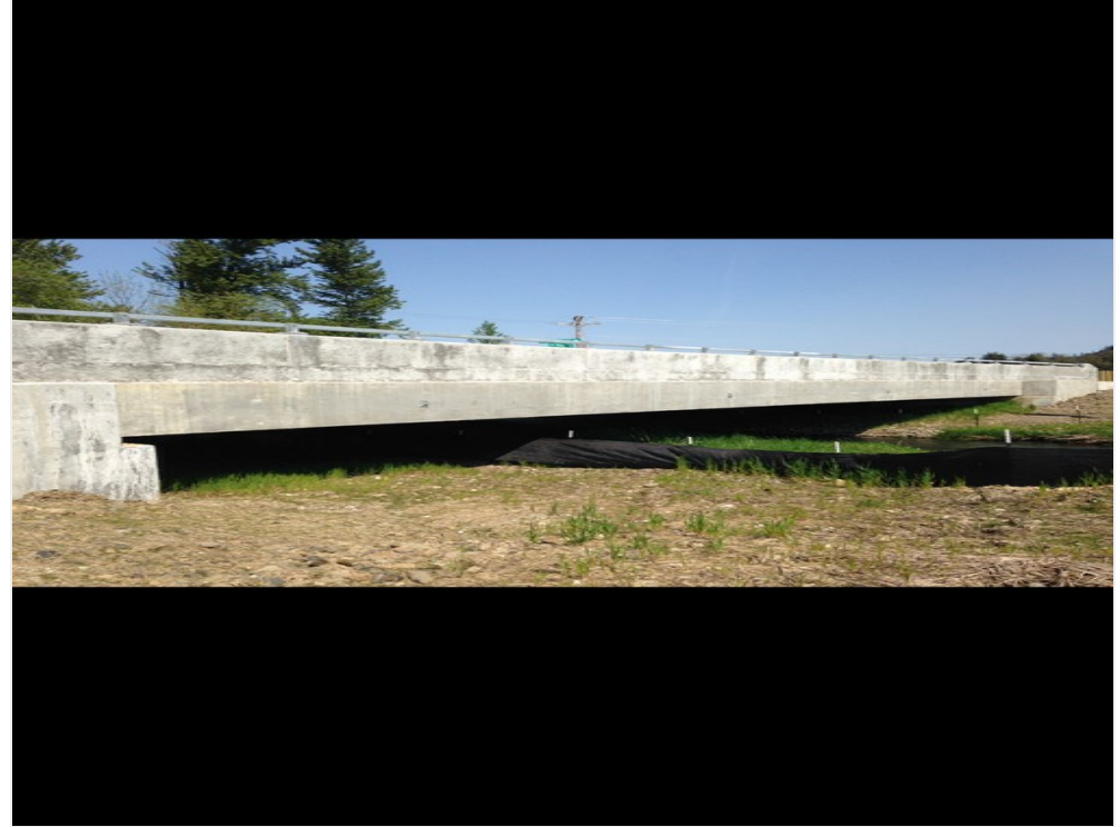
Increased Clearance with New Mill Creek Bridge
