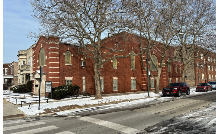
CHURCH EXTERIOR VIEW FROM 70TH STREET
