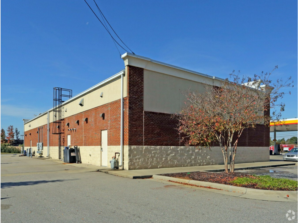
Back of Building
