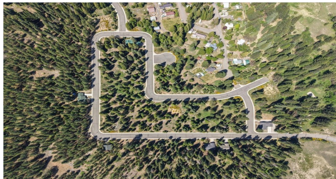
Aerial — completed road network
