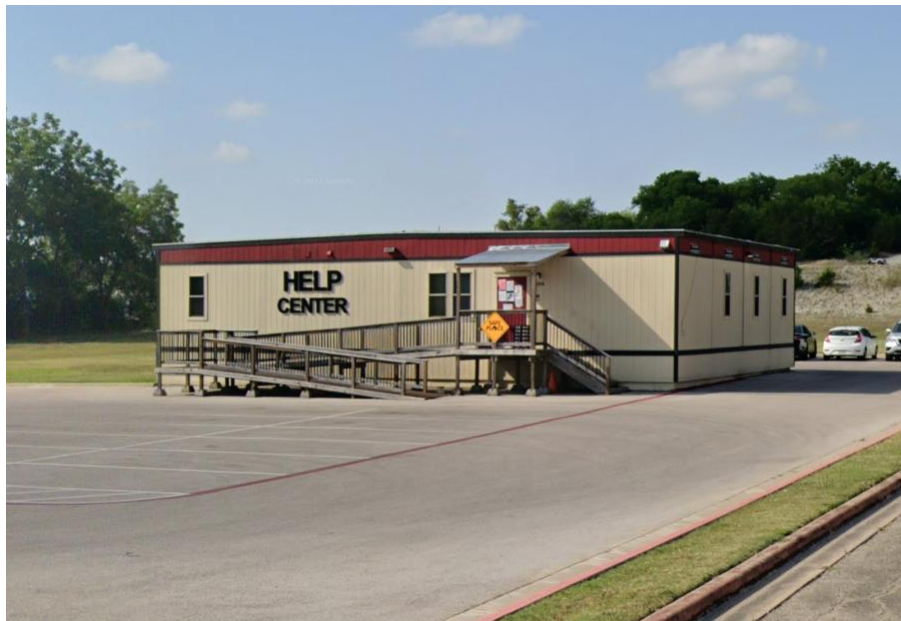
170391 Building 204 Exterior photo from Google Street View
