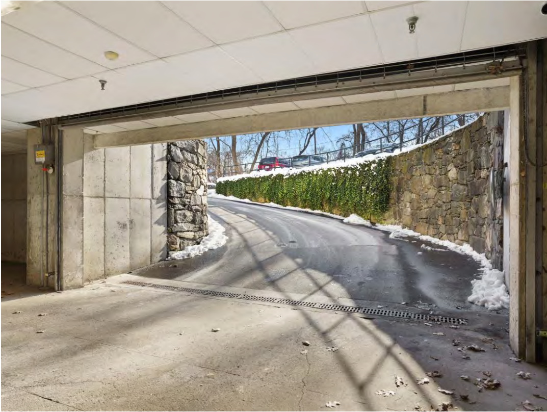
Indoor Underground Garage Entrance
