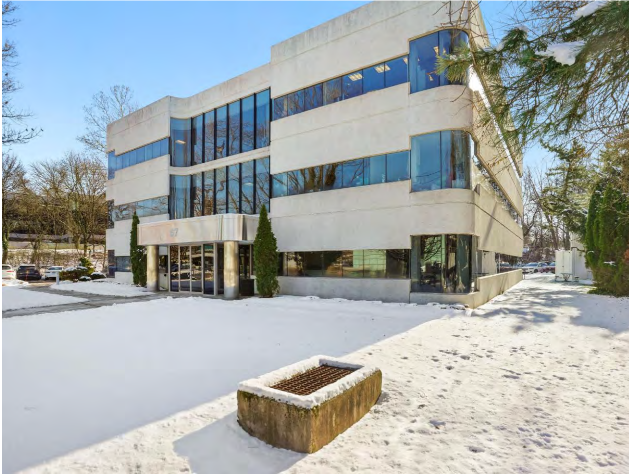
Exterior of Building
