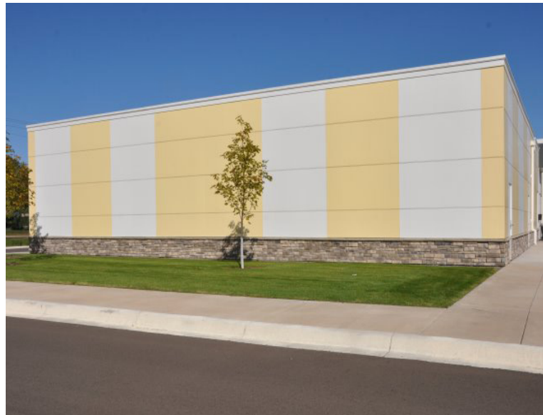
South Side of Building
