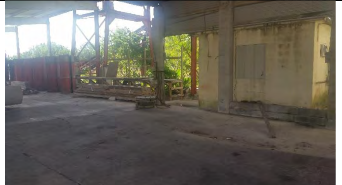
Photograph 22 – Typical view of the concrete production area
