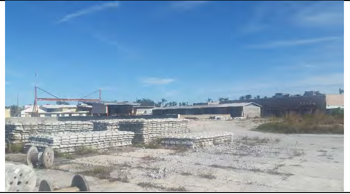
Photograph 10 - View of concrete debris located on the southwest portion of the subject site
