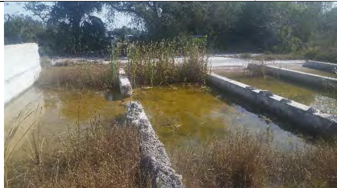
Photograph 13 - View of the wash water system on the southeast portion of the subject site
