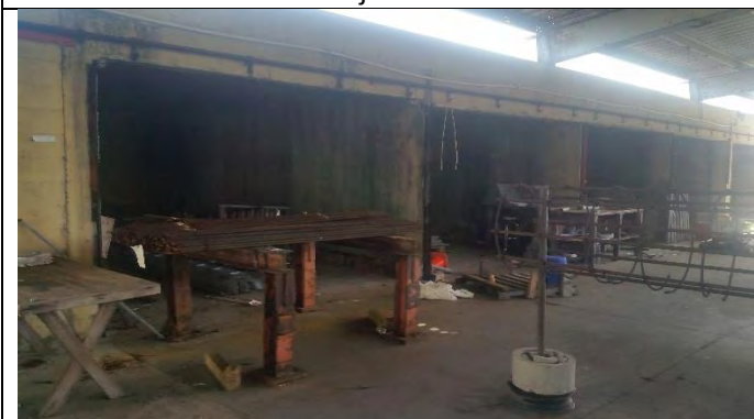
Photograph 23 - Typical view of the concrete production area
