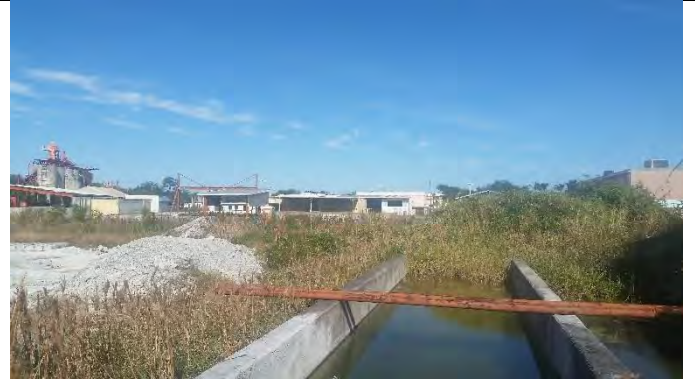
Photograph 12 – View of the wash water system on the southeast portion of the subject site
