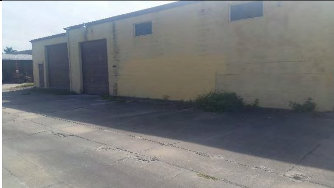
Photograph 29 – View of the office/storage building located on the north central portion of the subject site
