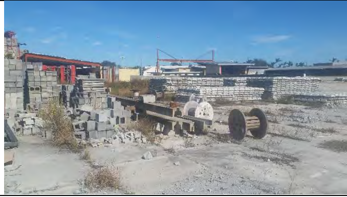
Photograph 9 – View of concrete debris located on the southwest portion of the subject site
