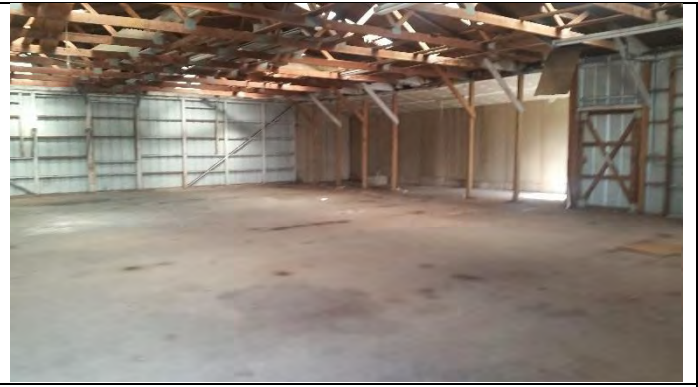
Photograph 34 - View inside storage building located on the subject site
