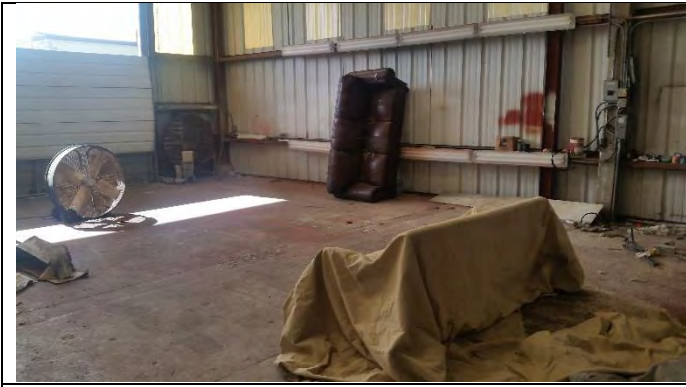
Photograph 33 – View inside storage building located on the subject site
