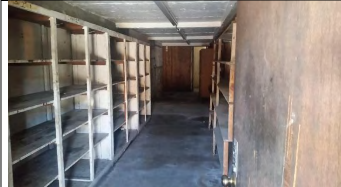
Photograph 21 – View of storage area within building on subject site
