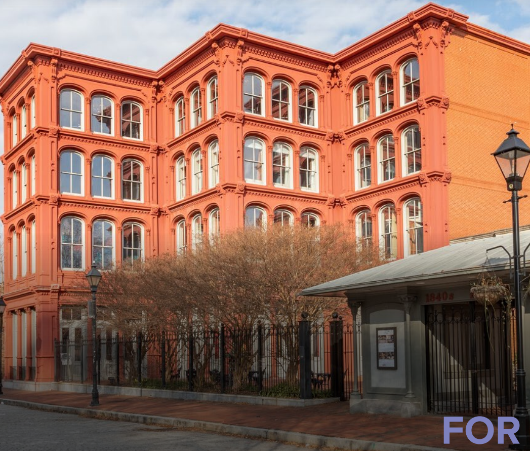
FAVA BUILDING & WAREHOUSE BALTIMORE, MD 21202
