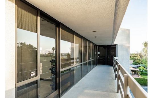
Exterior corridor entry
