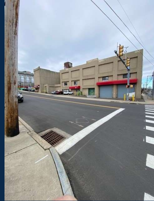
Front of Building
