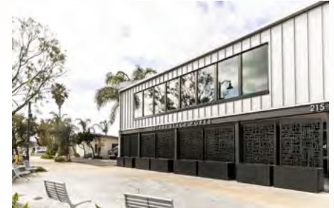
EXTERIOR PATIO FOR SUITE 100
