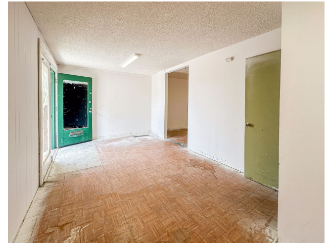
UNIT A2 — REAR ROOM
