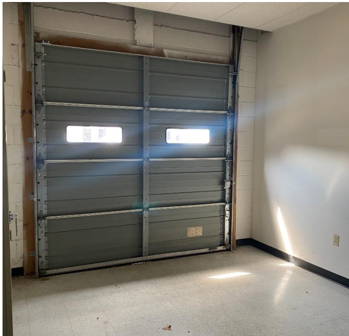
Dock Area (Inside)
