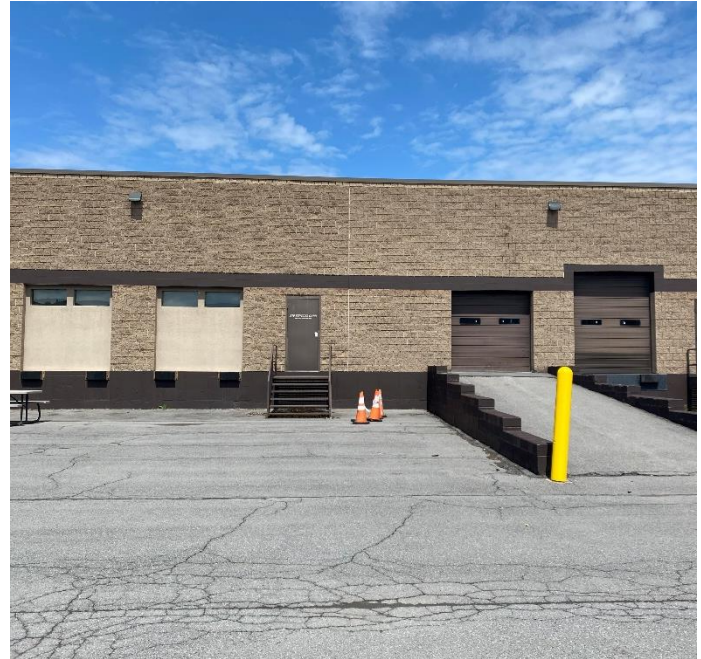
Dock Area (Outside)
