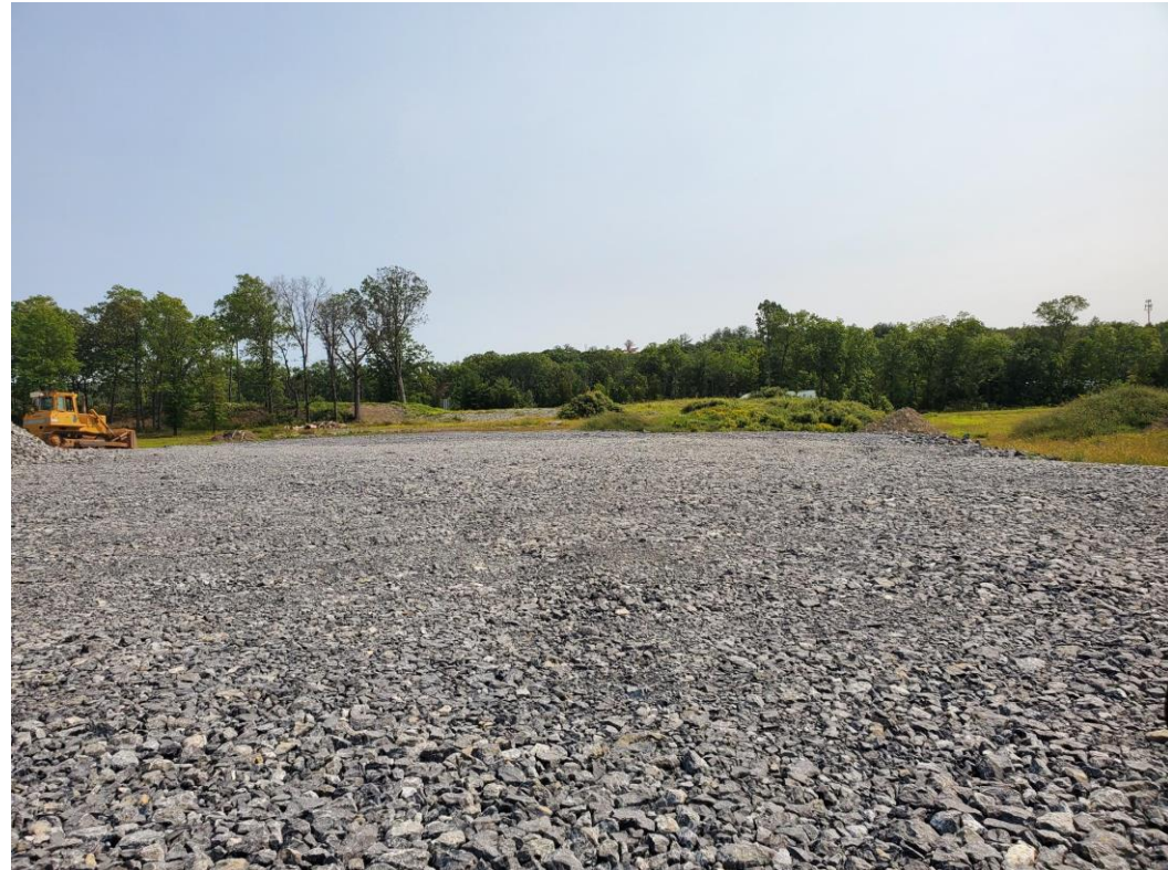
Site at rear
