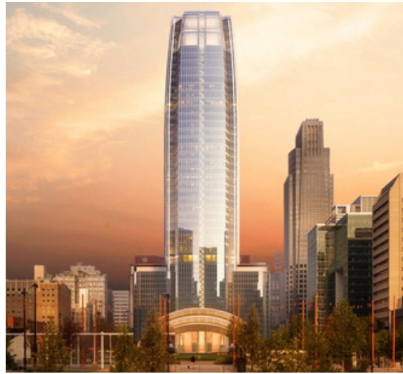
MUTUAL OF OMAHA TOWER: Mutual of Omaha is currently developing one of the tallest buildings in the region. The $600M 44-story glass tower stands at a staggering 677 feet.
