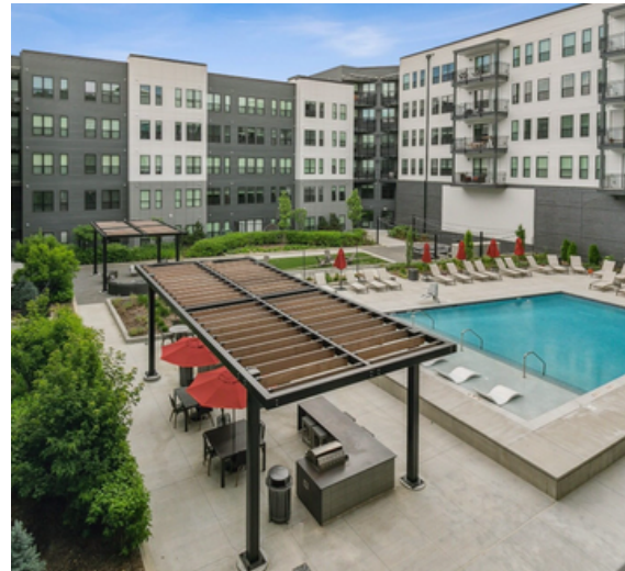
NEW APARTMENTS AND HOTELS: With downtown's recent developments, many residents are relocating to this area. Over 1,500 apartment units have been added in the last few years or are under construction. Along with over 450 hotel rooms in development
