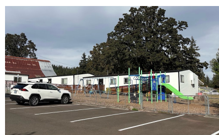
PARKING LOT RESTRIPTED (2026)
