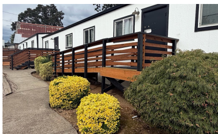
RAILINGS RECENTLY RENOVATED (2026)
