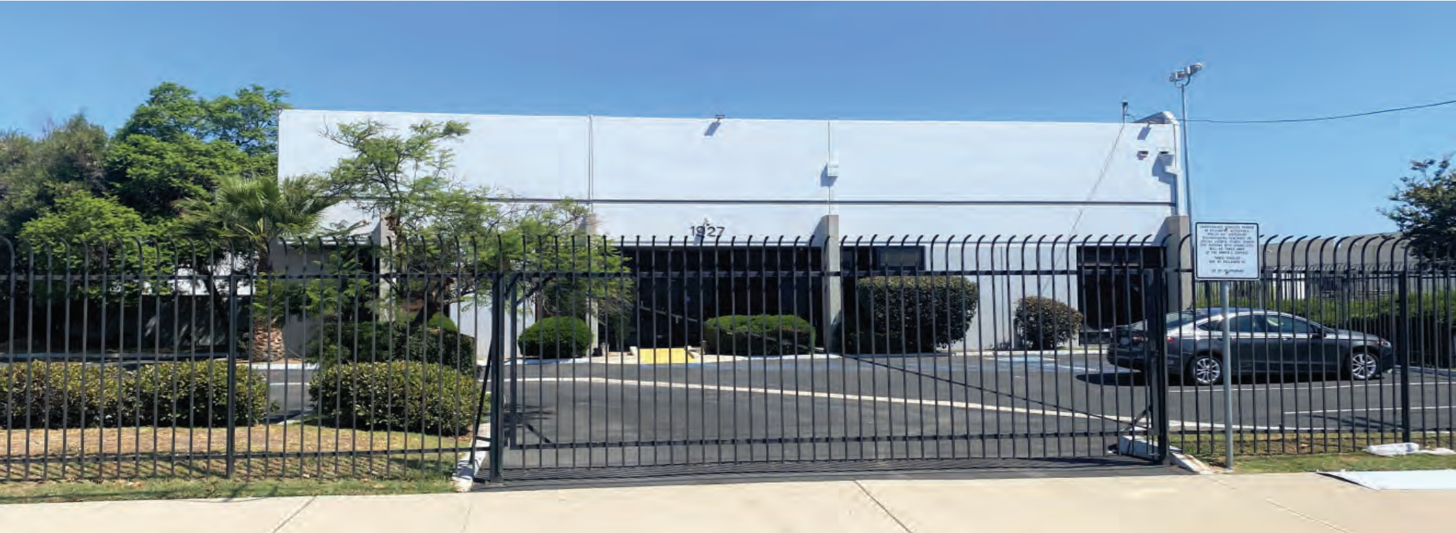
BUILDING PHOTOS | WAREHOUSE EXTERIOR
