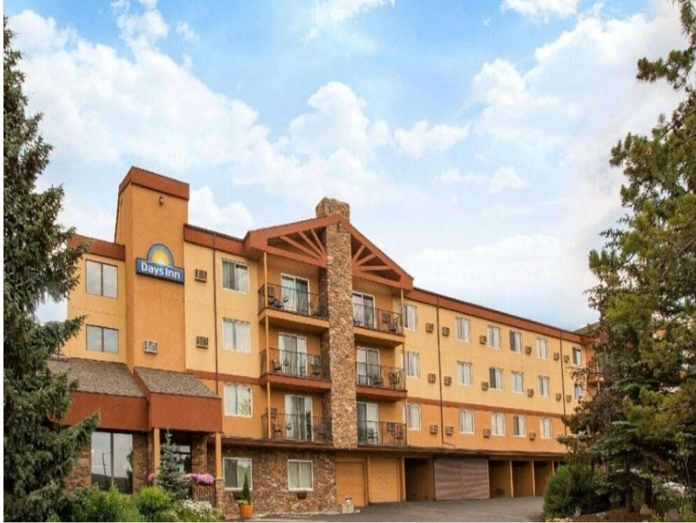
Front of Building
