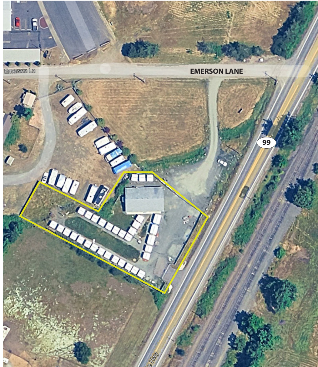
FORMER PALLET SHELTER HOUSING SITE
