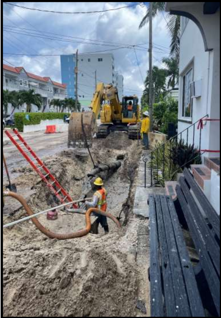
Excavation for pipe installation
