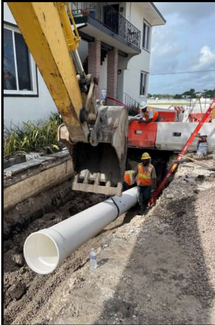
Stormwater pipe installation
