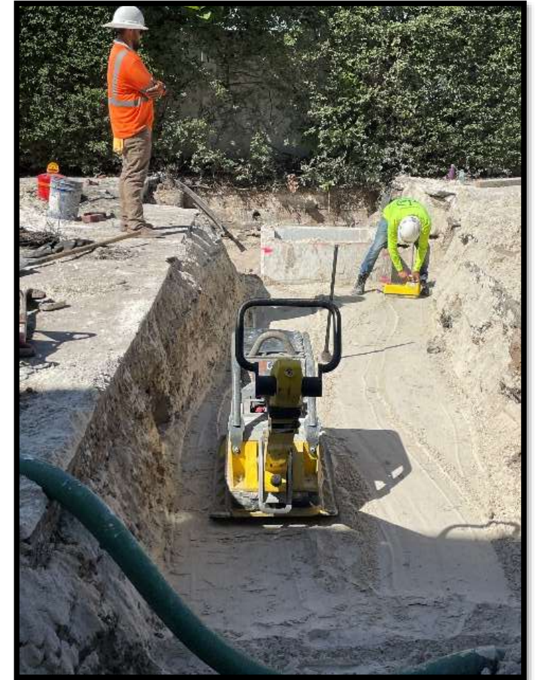
Compaction and testing
