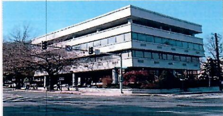
Exterior of Building
