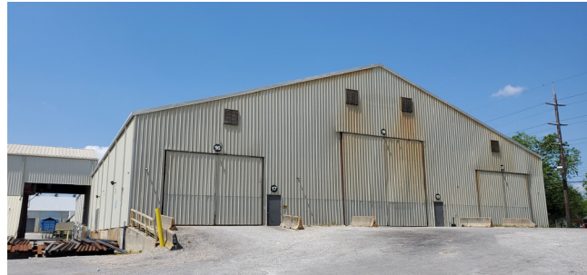
EAST-WEST CRANE BAY DOORS
