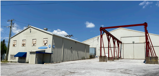
NORTH-SOUTH CRANE BAY, SHIPPING / RECEIVING OFFICE
