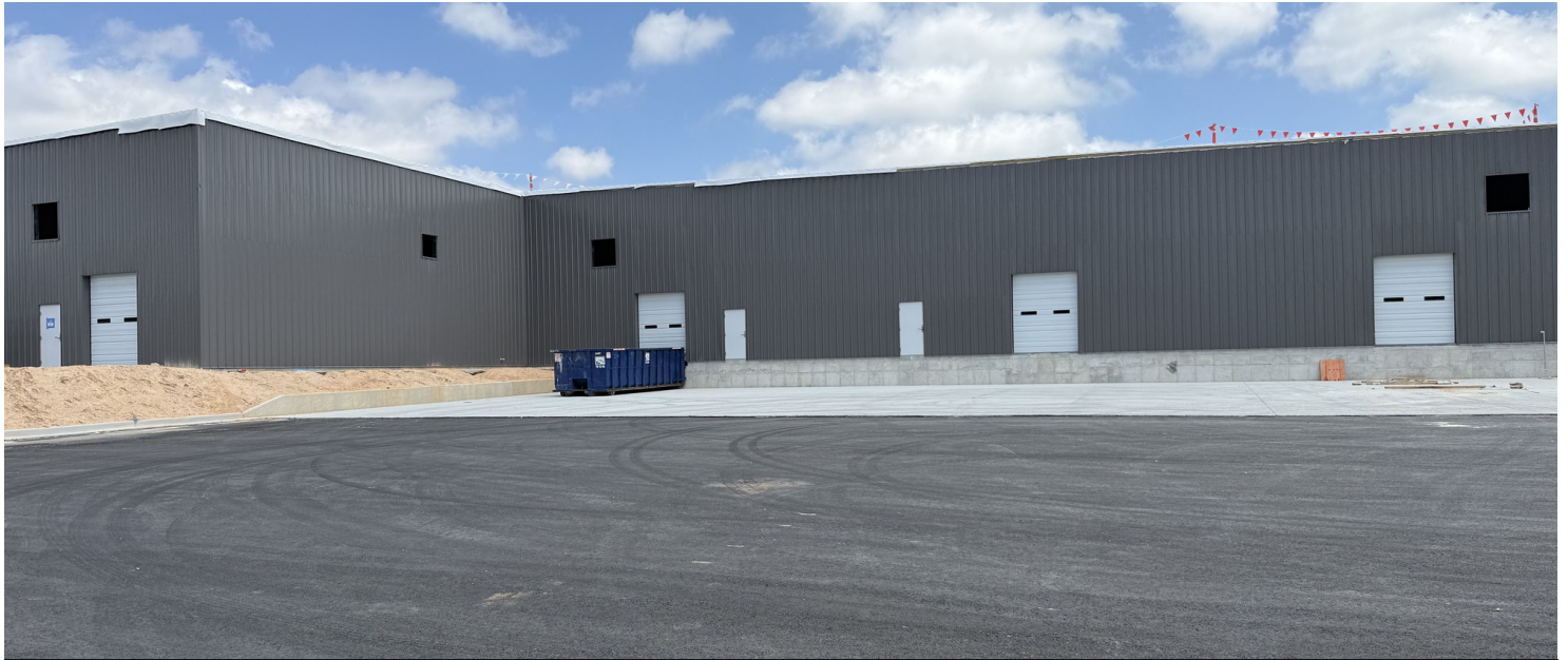
Construction in Progress 5-20-2026
