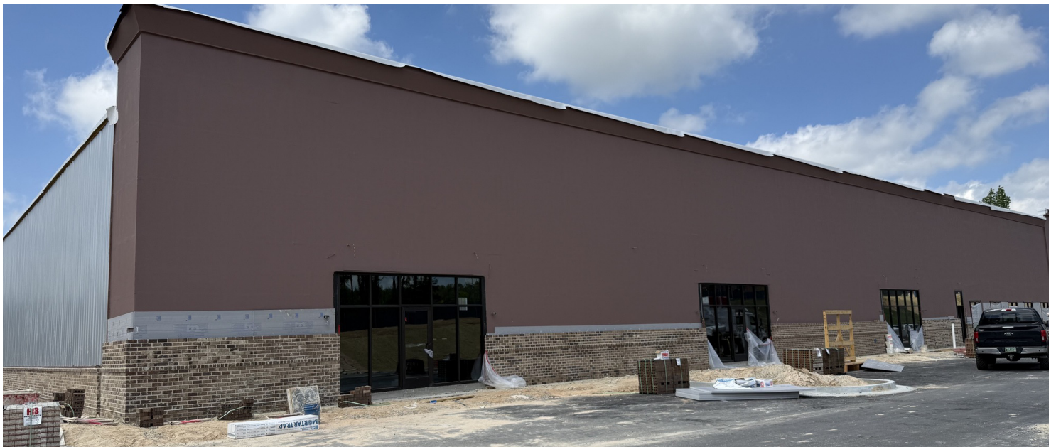
Construction in Progress 5-20-2026
