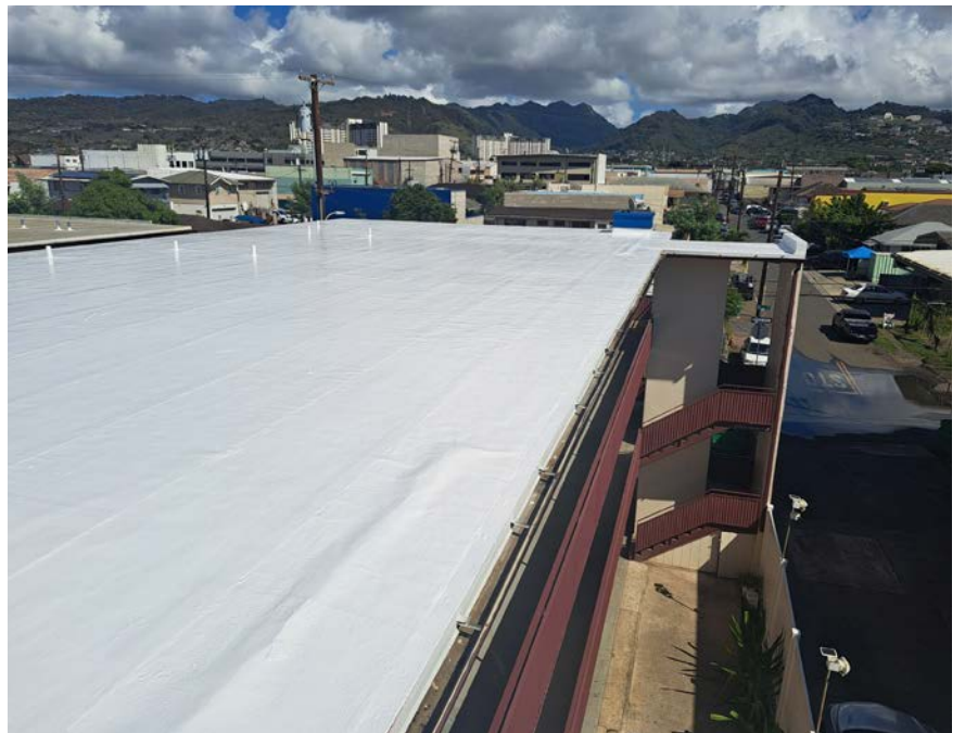
New Roof (Nov. 2022)
