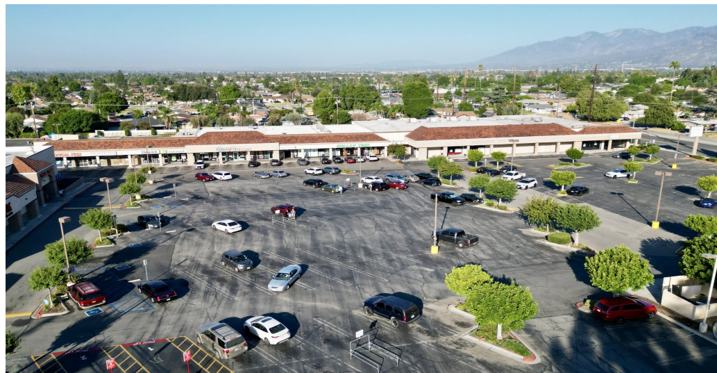
Unit 1071 - Aerial with Unit 1071 on the Right
