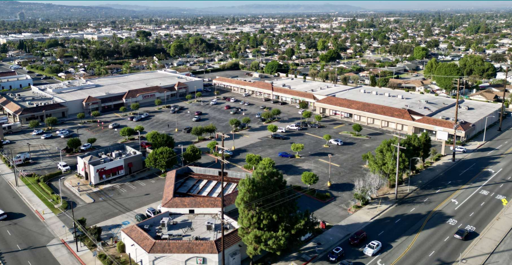
Unit 1071 - Aerial End-Cap at 8,063 SF
