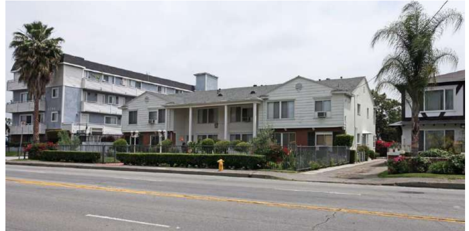
E 5330 Whitsett Ave North Hollywood, CA 91607
