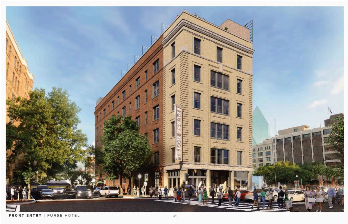
Purse Building | 601 Elm Street, Dallas, TX
