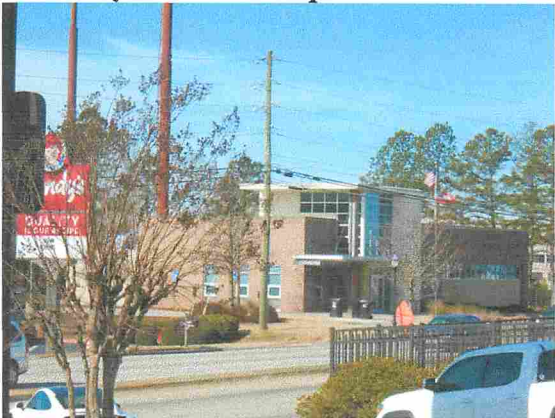
New City Police Headquarters
