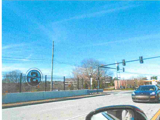
Mid-rise office in SWC of I-85 & Ga 317
