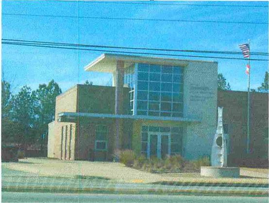
New City Police Headquarters
